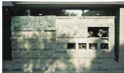
The Four Seasons mural The Four Seasons Bldg. Tiana, Spain
